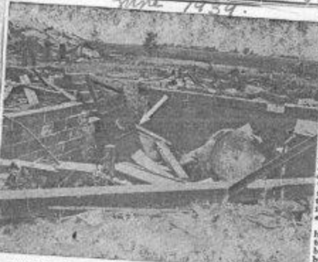
View of the basement at the James Cooley farm. The family of three died in the basement just as the storm struck and were saved from possible death or serious injury by the trap door, indicated by arrow, that flew into the basement, breaking and splintering several boards of the door. They were coddled under the door at the point indicated by arrow.
