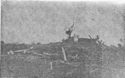
THERE WAS A HOUSE —Until Saturday night's wind-storm took things into its own hands and here is the spot of rubble and splinterings that marks the last resting place of Omer Rough's house. There is not enough left now to make a shelter for a small car.
