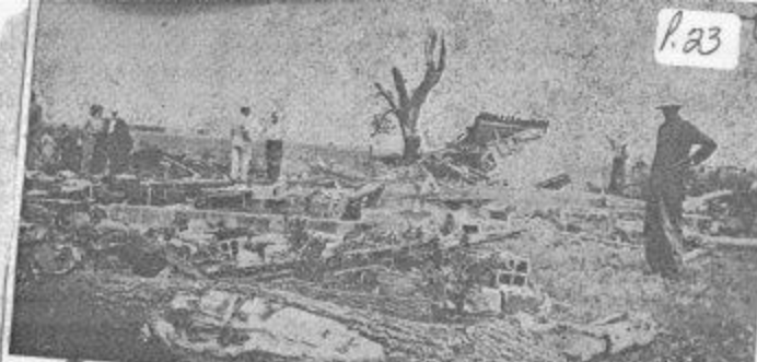
View of the ruins at the home of James Cooley, two miles southwest of Rash. The 14-room house was lifted from its foundation and completely demolished. Part of it can be seen in a pile near the site of what was once a large shade tree. Mr. and Mrs. Cooley and two children escaped building on this farm was swept away.
