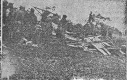
WANDERING HOME —This is the biggest pile of shattered lumber that was left in fields a half mile east of the Burley farm home foundation shown second from left this column. The scene is east of Brook, Indiana Sunday after some of the first shock had worn off.
