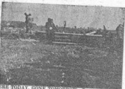
HERE TODAY, GONE TOMORROW —So say the women who look over the spot where the foundation is all that is left of the Burley farm home and farm buildings, 3 miles south of Brook. This farm house was blown into bits over a mile course northeast.
