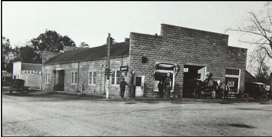
Original Building – G & E Christenson Garage
