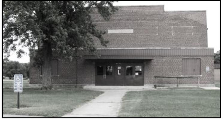
Lake Village Grade School Gymnasium
