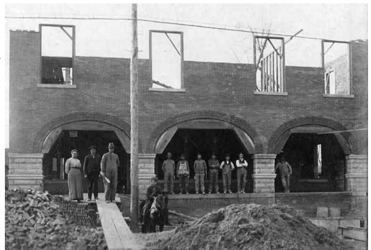
Building in progress, 1909, Sarah and the Don Brothers on the left; building crew standing under the arches of the hotel.
