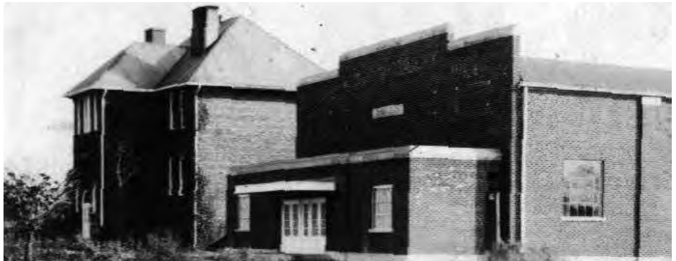
The new Lake Village Gymnasium was dedicated in 1939. The school today, Lake Village Elementary is utilized as part of the North Newton School Corporation.
