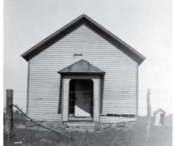
The school served the children in the northeast part of Washington Township 1907-1924. A map and list of teachers can be found at www.ingenweb.org/innewton .
