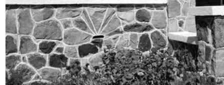
Floral designs of stone are found throughout the facade of the Arnold house.
