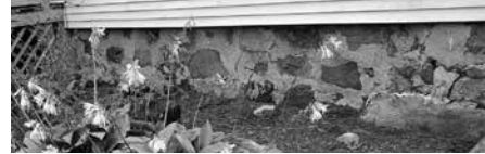
A home in Goodland has a fieldstone foundation as do many in Newton County.
