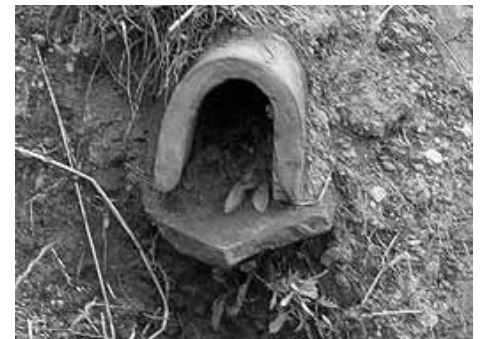
"U" shaped tiles used as field tile.
