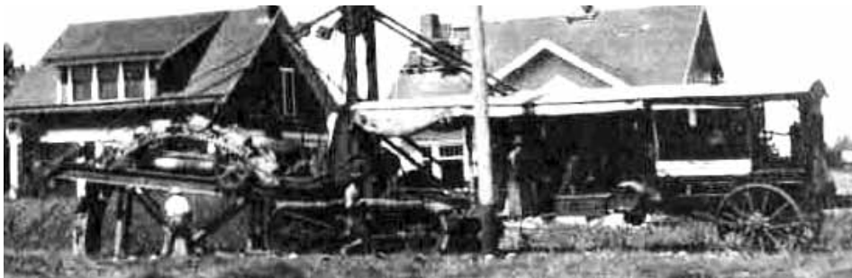
Typical 1920s steam ditcher, the likes of which were used in Newton County.
