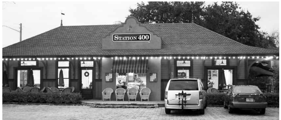
Top: A photograph of kids in the Kentland Grade School playground in 1958 shows the old NYC depot that stood in the northwest corner. Bottom. The NYC Depot as it stands today in Sarasota, FL, as the Station 400 restaurant. Photos courtesy of Dean Ford.
