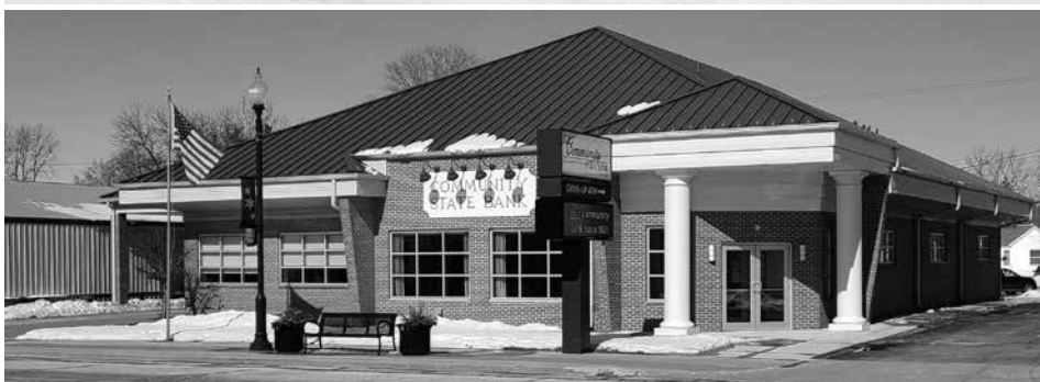
Top photo dated 2015, bottom 2021 of the Community State Bank in Brook.
