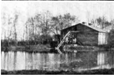
Top, home built 1898, standing 2021; bottom, Stewart's Ice Plant circa 1916.
