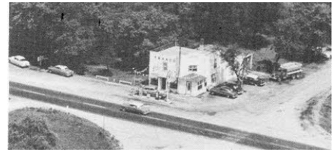
Texaco Station, US 41 (one-lane) and SR14.
