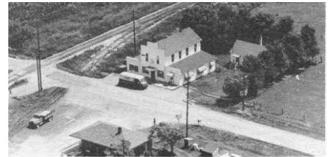
Enos Store, note railroad spur to elevator.
