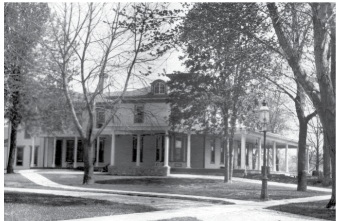
A rare view of the second NuJoy back in the day - looking northeast to the west side of structure, when it appeared as the home of AJ Kent.
