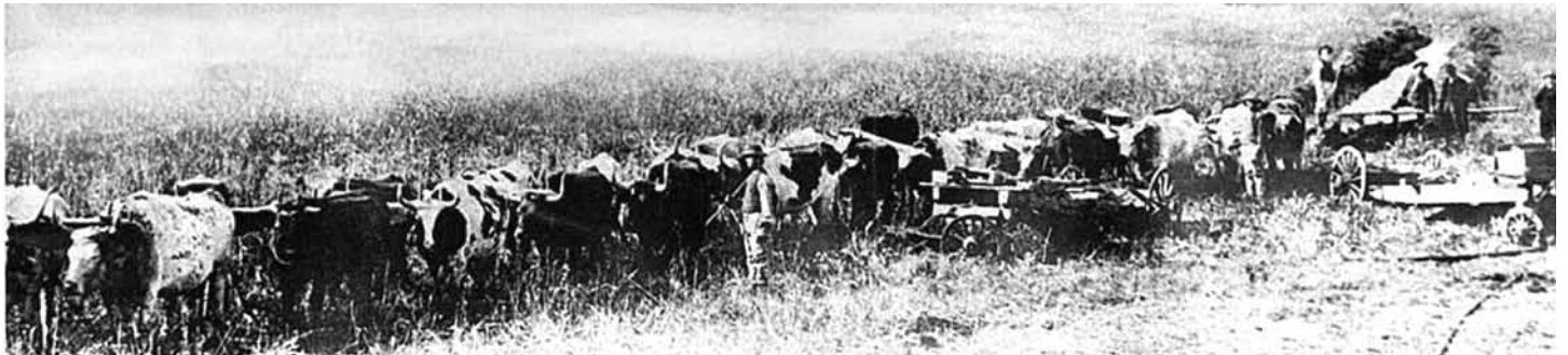
An ox-drawn ditching machine similar to this one used to dredge the ditches in Iroquois County, Illinois, may have been used to cut the original Beaver Lake ditch, and complete the final cut in Newton County. Photo reprinted from the Illinois Steward, Summer, 2007.
