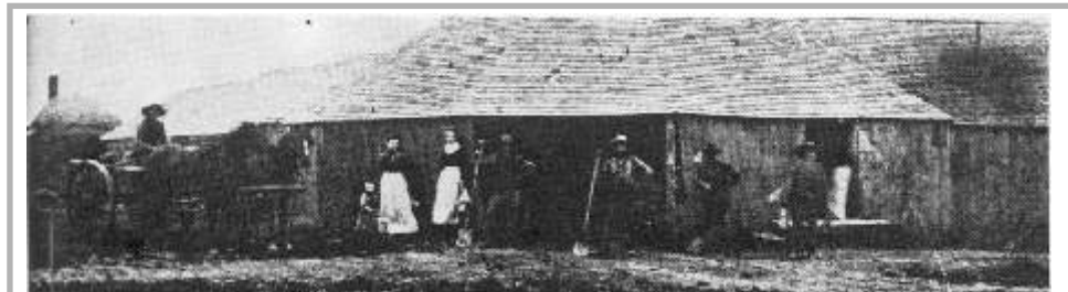
Mt. Ayr Tile Factory, owned by Coovert and Stucker.
