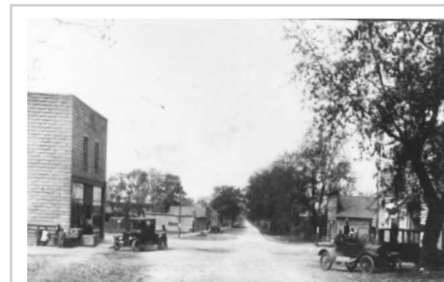
A scene from Lake Village, looking west from the main intersection of town. Submitted by Gerald Born
