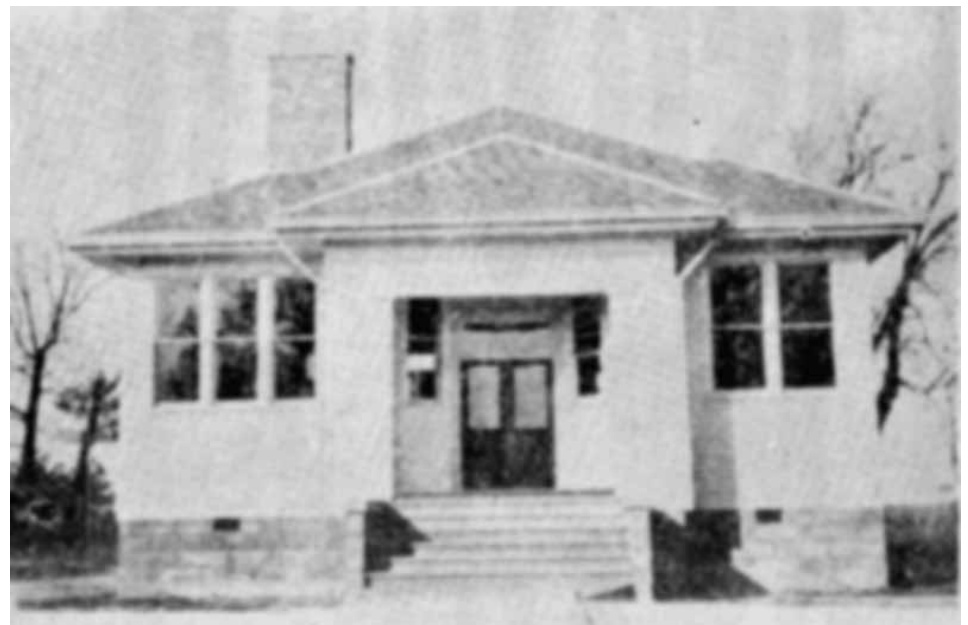
Original school structure that burned.1915.
