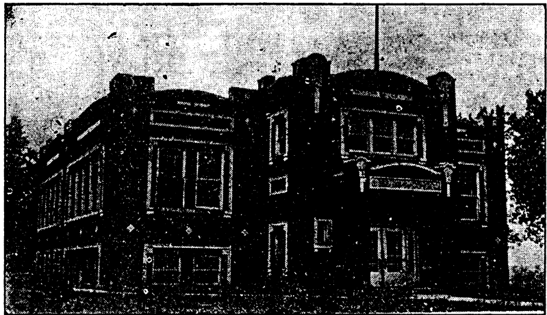
ROSELAWN CONSOLIDATED BUILDING
